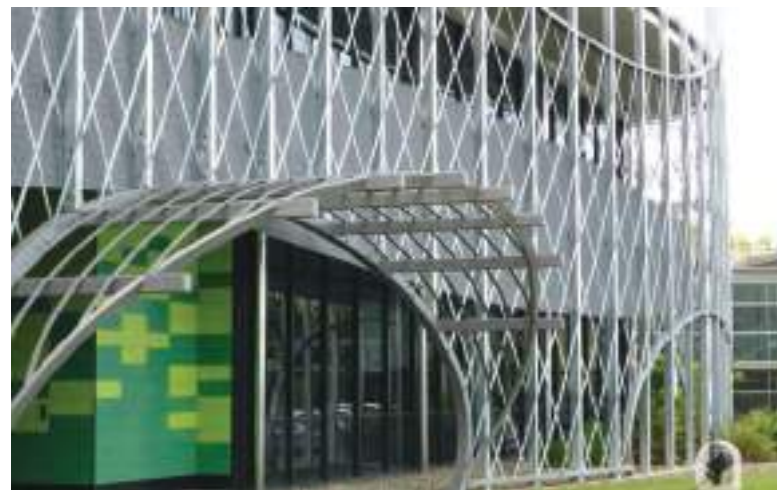
Here the hot dip galvanized trellis combines with a modern skin to complete the building entrance.
