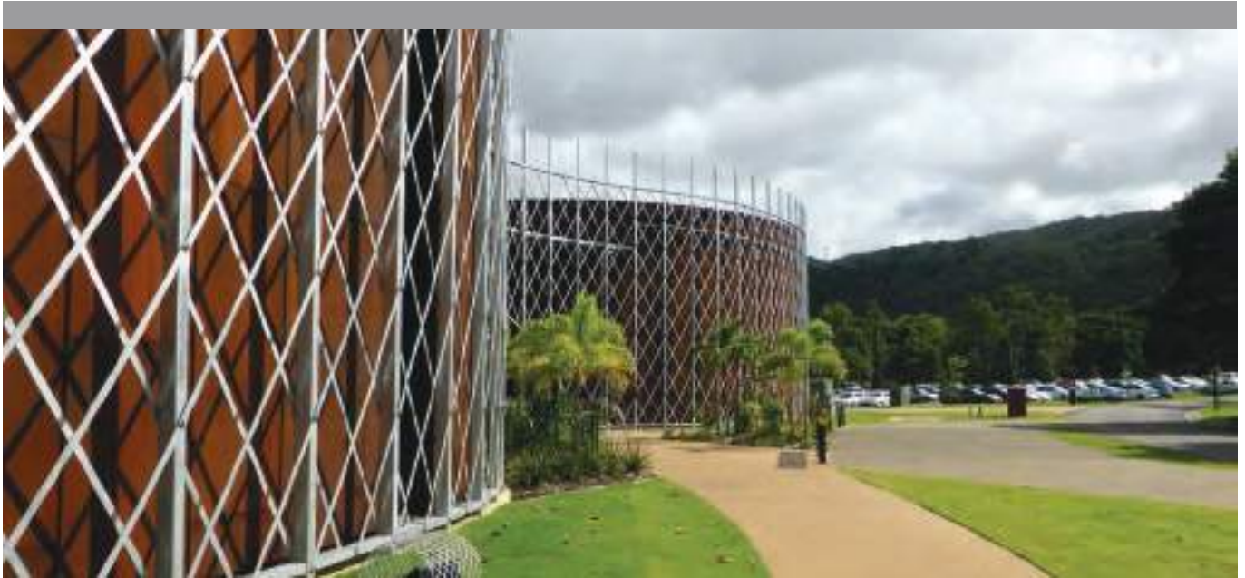
Hot dip galvanizing and weathering steel combine to provide a stunning contrast clearly visible from the nearby main road.
