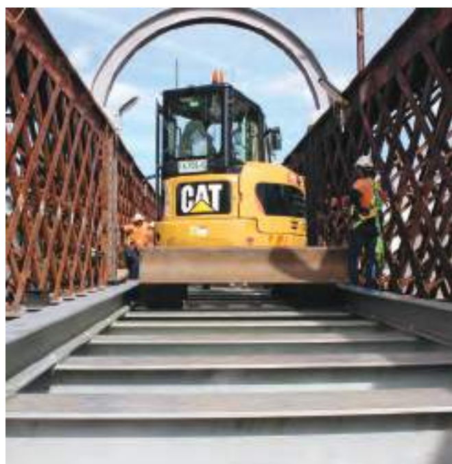
Galvanized stringers being secured to the newly-installed cross-braces.
